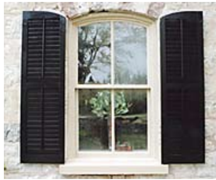
Contrasting black wooden louver style shutters with curved top provide a good fit for the window.
