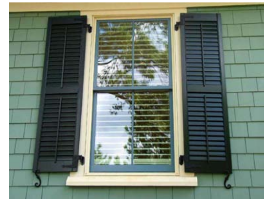
Proportioned shutters with functioning hardware. Note shingle walls.
