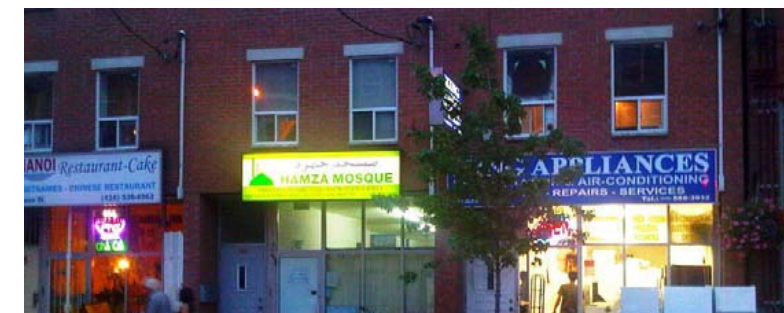
Signs fabricated from Plexiglass, are back lit, not integrated into the architecture of the building and have little appeal to a consistent theme.
