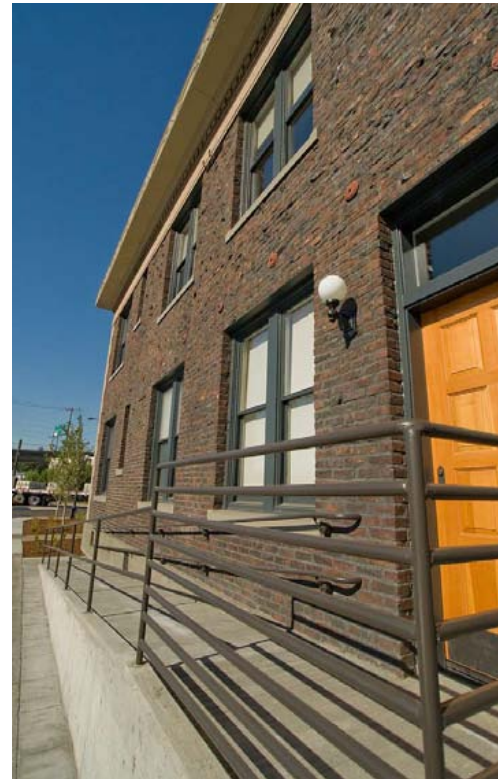
Concrete ramp with guardrail provides access to historic building. Note colour of handrail.
