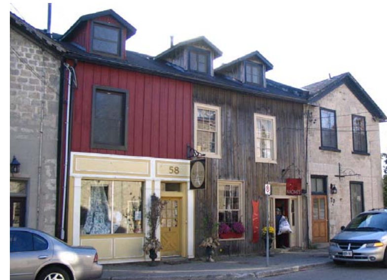
Two storefronts within one architectural framework. Lack of unified appearance.
