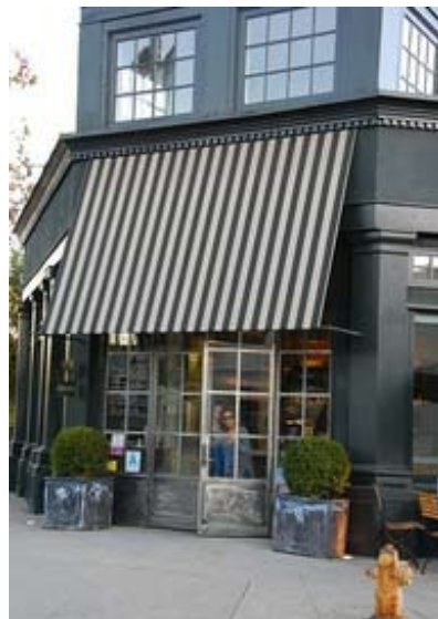
Acceptable awning alternative; steep pitch may respect sight lines on street corner or screen unsightly building face.
