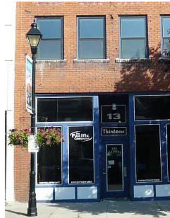
Building entrance flush with sidewalk - barrier-free
